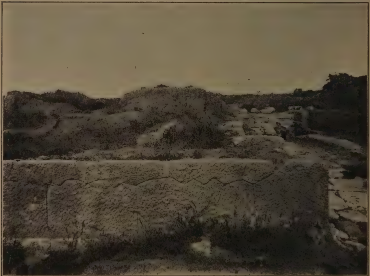
FIG. 19. — Notched masonry at Eretria.
